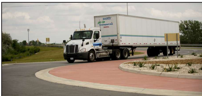
Figure 3-15. Large truck using truck apron on roundabout.
