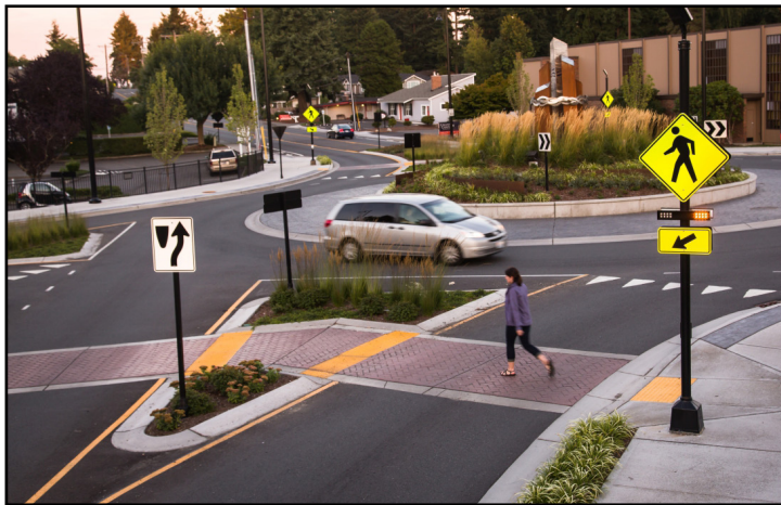
Figure 3-14. Accessible Pedestrian Crossing
