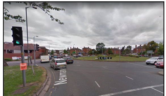
Figure 3-6. Signalized roundabout in United Kingdom.
