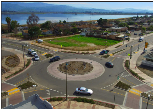
Figure 1-9. Roundabout in Woodlake, CA
