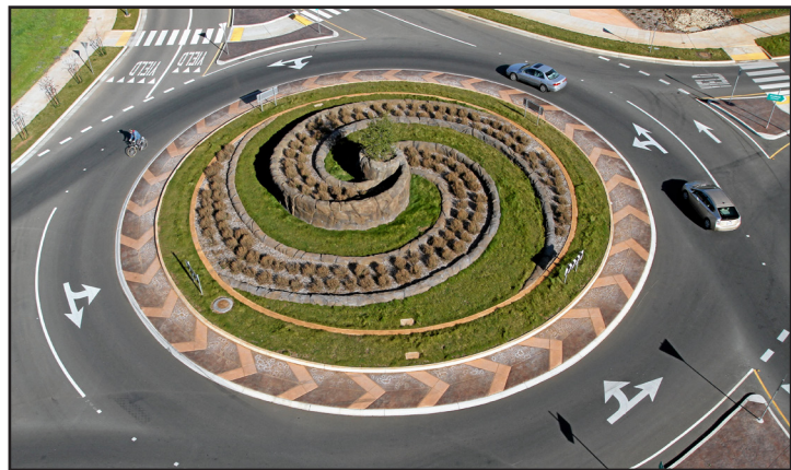
Figure 3-22. Elaborate roundabout landscaping in Chico, CA
