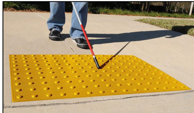
Figure 3-20. Truncated dome on sidewalk ramp.
