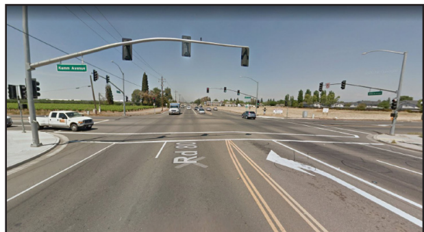
Figure 1-6. S. Alta & Kamm Ave, looking north. Source: Google Earth 2019
