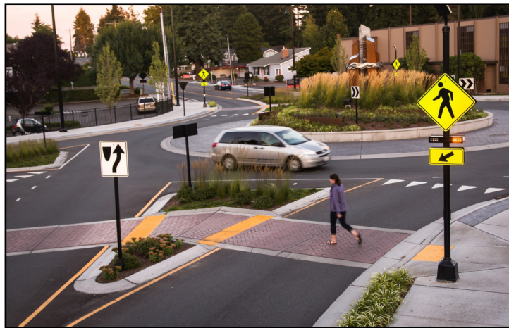
Figure 3-14. Accessible Pedestrian Crossing
