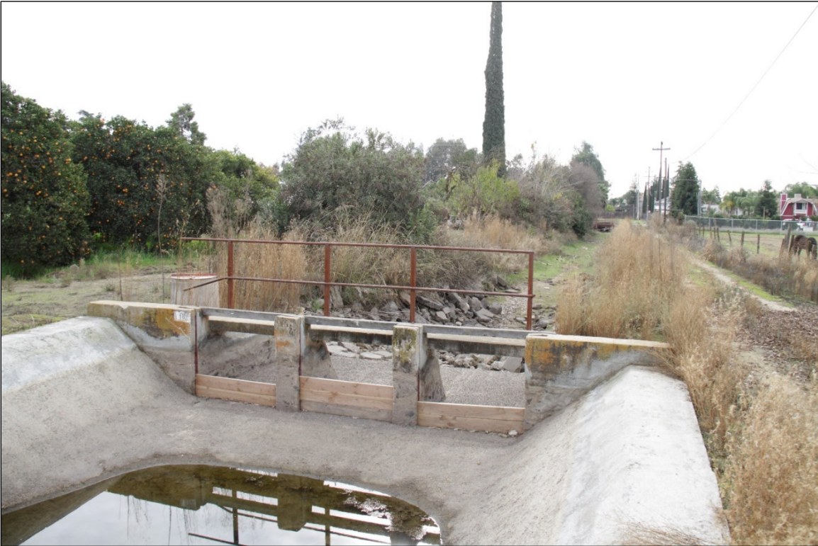
Figure 5 Dinuba Town Ditch; view to the south.
