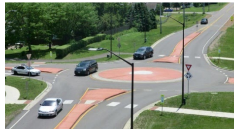
Roundabouts (E:3, C:3, IC:3)
