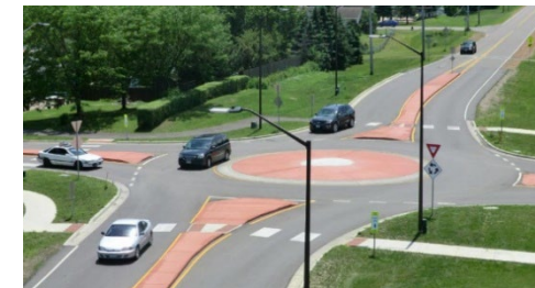
Roundabouts (E:3, C:3, IC:3)
