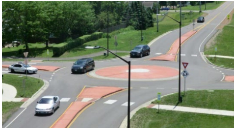
Roundabouts (E:3, C:3, IC:3)
