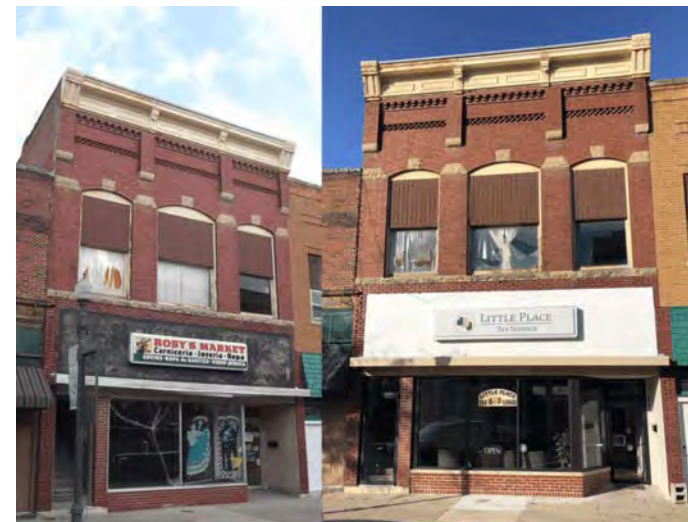
Image 1-3: Renovation of an existing building to match historic architecture.
