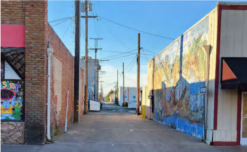
Figure 6-30: Existing Conditions of Pilot Alleyway at 135 E Tulare St.
