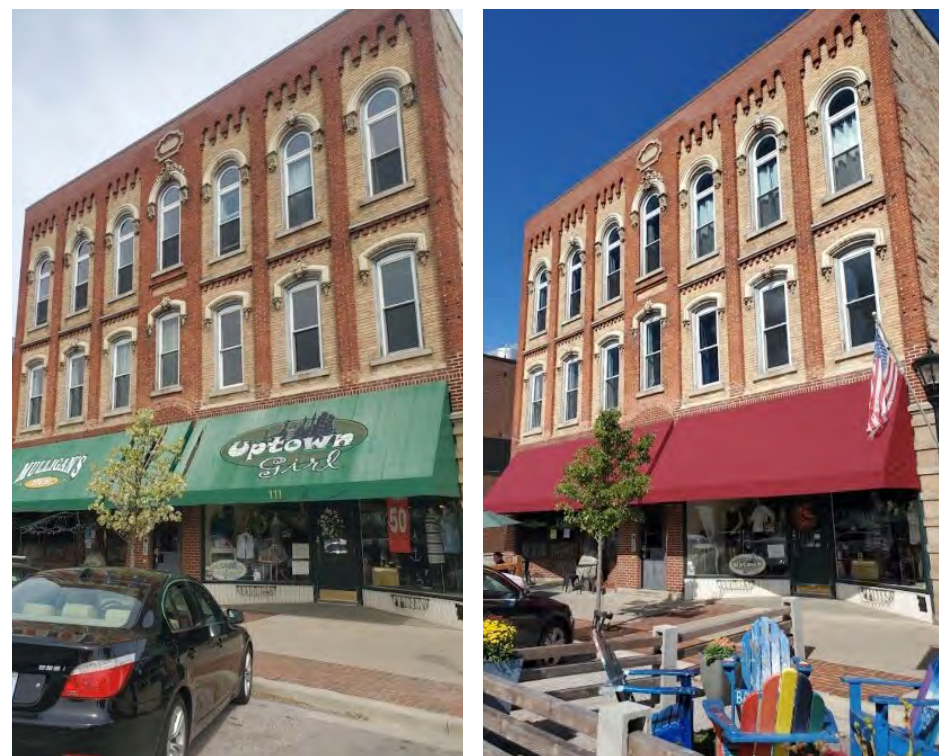
Figure 1-5: Before and after a façade renovation in downtown Bay City.
