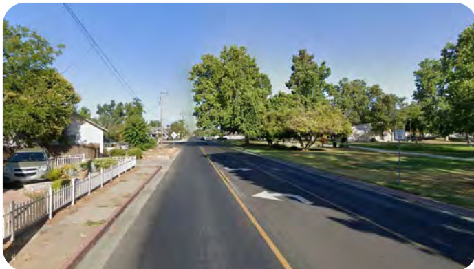
Image 3-3: El Monte Way Lacking Sidewalks
