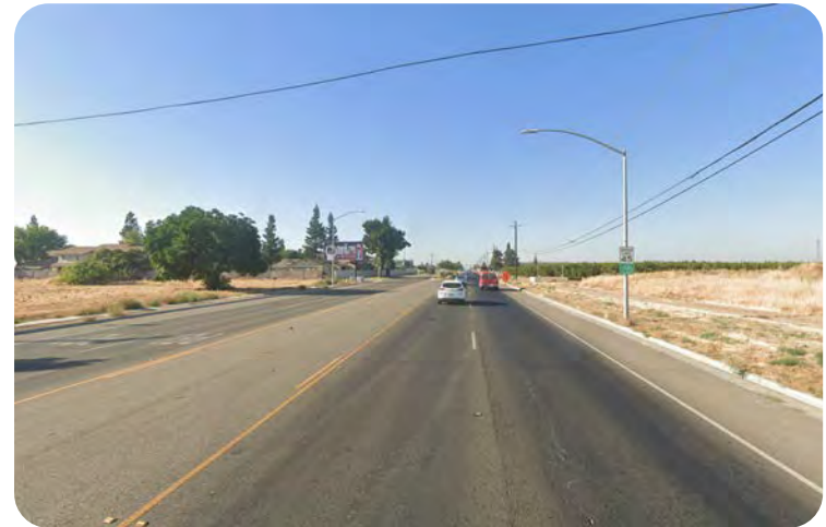
Image 3-2: South Alta Avenue Bike Lanes
