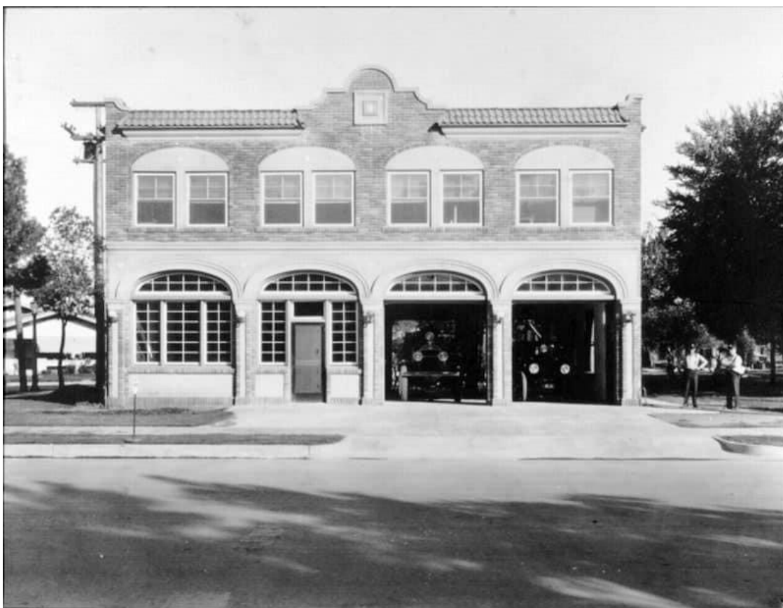
1920 Dinuba Fire Station
