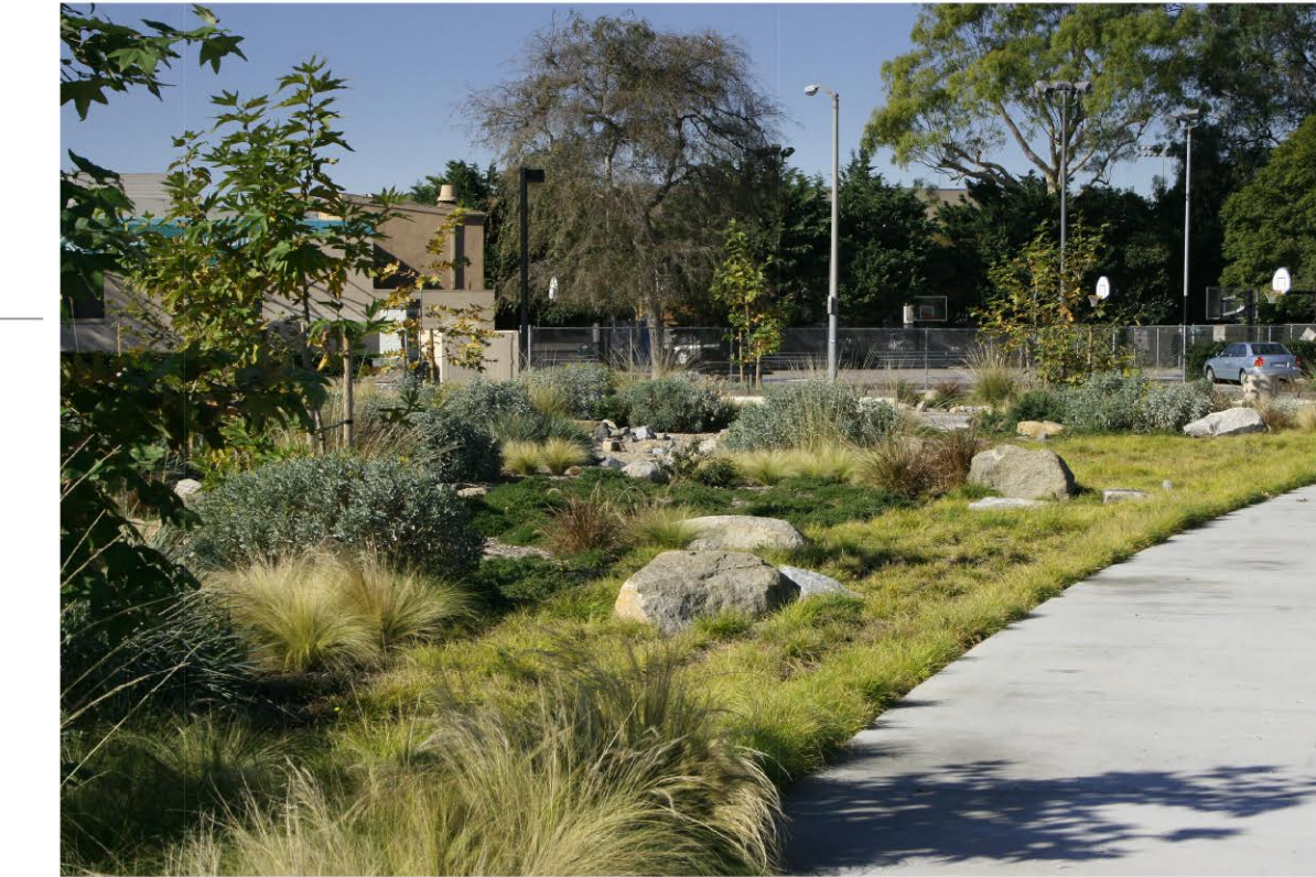
WATER DETENTION BASIN
