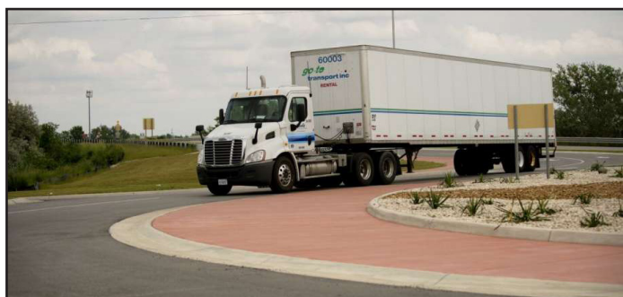
Figure 3-15. Large truck using truck apron on roundabout.
