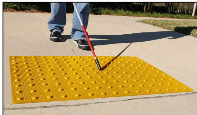
Figure 3-20. Truncated dome on sidewalk ramp.
