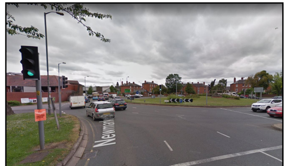
Figure 3-6. Signalized roundabout in United Kingdom.
