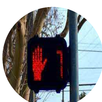
Install Pedestrian Countdown Signal Heads
